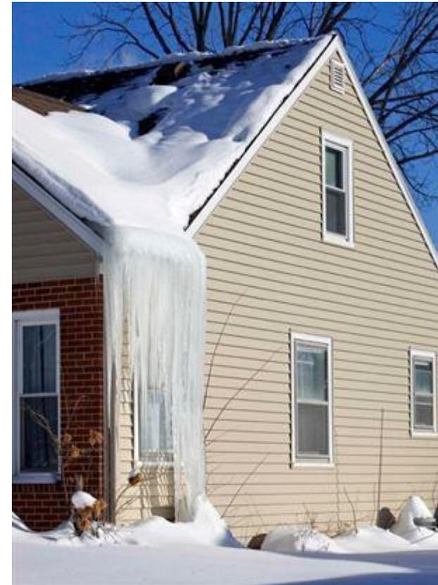
Leaf guard is just that; a system to prevent leaves from entering the gutter. Most leaf guards are a solid surface with perforations to allow water to flow into the gutter. The perforations must be small enough to keep debris out, but allow water in. These perforations freeze over quickly. Therefore, homes with leaf guard will see ice cycles more quickly than others. You may also see water coming over edges and off the sides of gutters where it normally wouldn't when the perforations are open.
