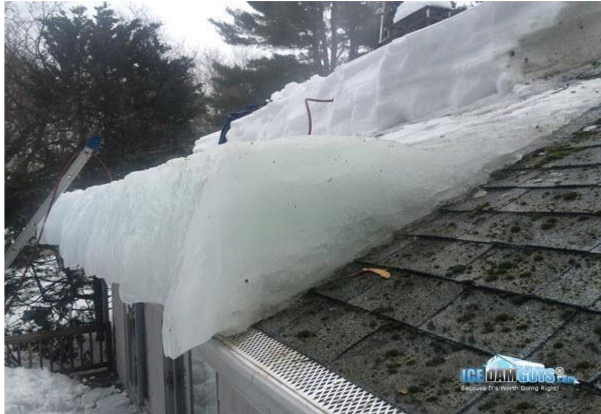
What is done to protect the home and stop ice from forming at the edge of the roof? Ice guard is applied at the eaves and valleys where ice and snow collect. Ice guard is installed up to a point that reaches above the freeze line. This protects the home from ice dams. Heat cables can also be installed that melt snow and ice away at the eave and gutters to give melting water from above an avenue to travel rather than being blocked. They do not eliminate all ice or snow, but they do help.
